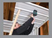
6 Begin the next row of steel panels installing the overlap rib onto the first panel installed. Fasten screws into the flat, next to each rib at every ceiling joist.
