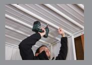
Install stitch screws into the overlapped rib 2' on center. This will attach the two steel panels together, creating a stronger ceiling liner.
