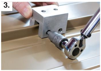
Tighten the set screws to a minimum of 50 in/lbs each using a calibrated torque wrench.
